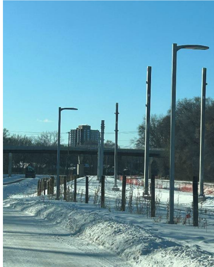
Final Overhead Contact System poles set, Minneapolis
