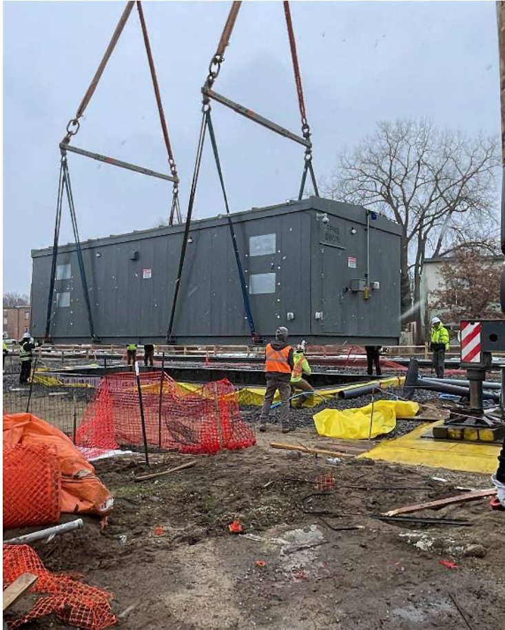
Setting of final traction power substation, Minneapolis
