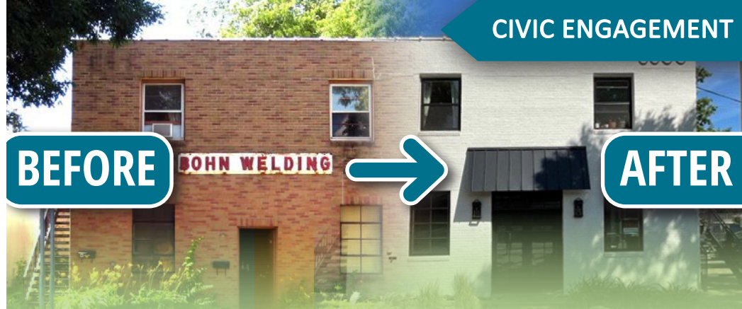
Improvements made by a St. Louis Park business using city grant funding.
